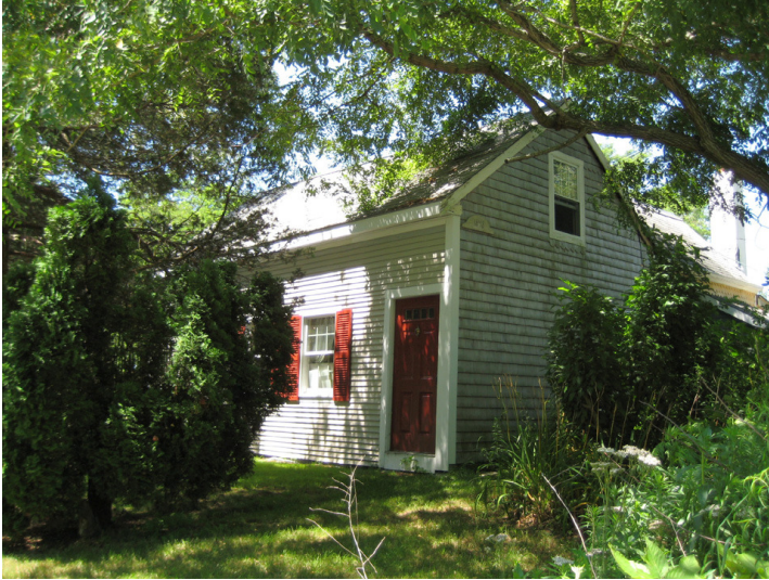
Southeast and northeast elevations
