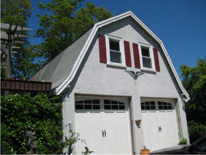
72 River Road Garage
