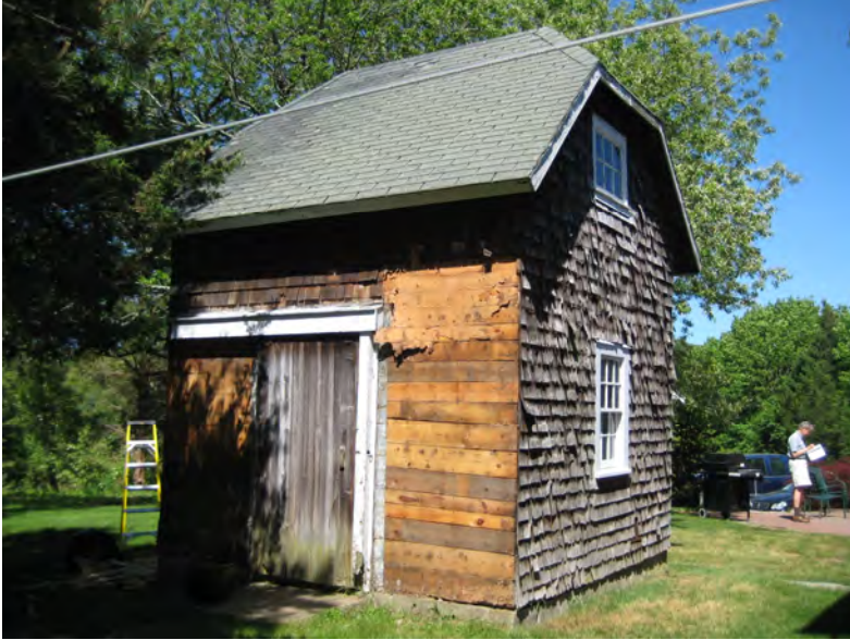
Bog Pump House (undergoing resingling)
