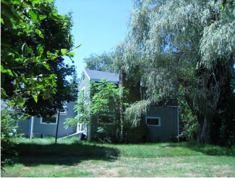
Northeast elevation showing fieldstone chimney
