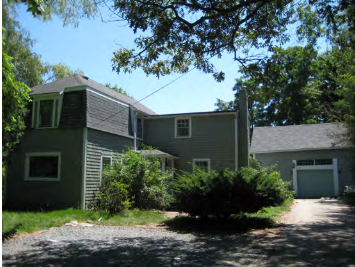
Northwest elevation with barn
