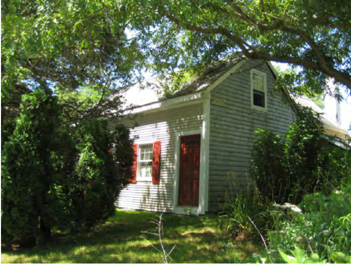
Southeast and northeast elevations
